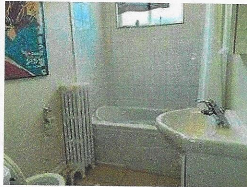
16 U: RENOVATED 4 Pc. Bathroom (2006)
